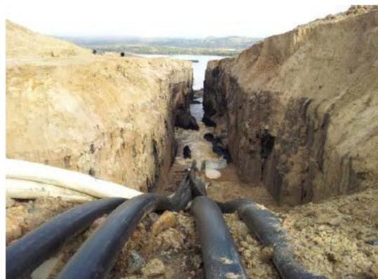
Figure 10. PE100 pipes used to dewater the mine
